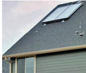
*Seattle Housing Authority installed a Baxi solar water heating system at High Point in March 2009. The system includes the solar-compatible Baxi Luna 3 Comfort combination heating and domestic hot water wallhung boiler, which is capable of accepting pre-heated water from the solar storage tank. The green building initiative should generate additional fuel and cost savings.*
